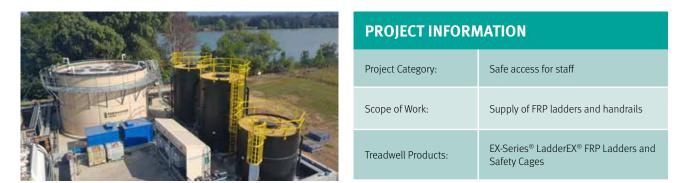
Our client undertook a complete mechanical plant design for a milk plant in New South Wales. This included three large tanks with top access safety platforms; this was to allow for easy installation and removal of large aerator mixers. Their design included ladders and ladder cages to provide safety to personnel using the roof mounted manhole access. These ladders also needed to be lockable to prevent non-permitted access.
