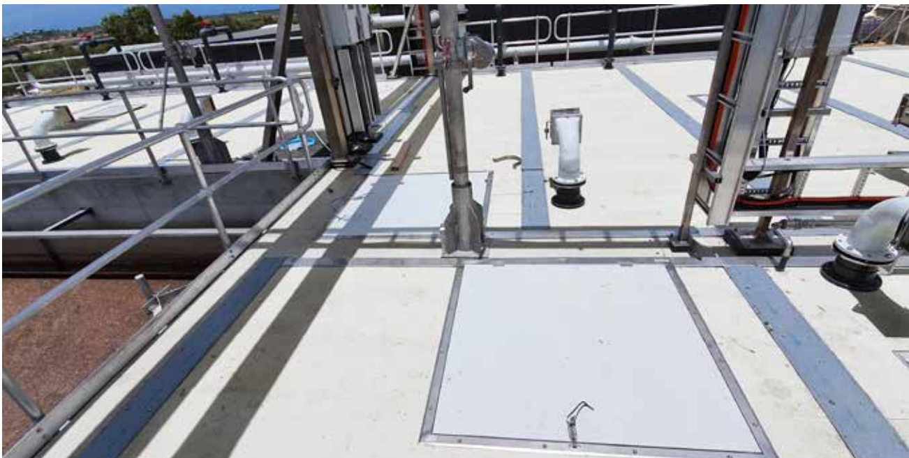
SureLine® Odour Cover Hatch. Queensland, Australia.
