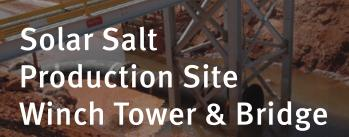
Particular attention had to be paid to the extremely corrosive environment the winch tower would sit in — this meant that the majority of conventional materials would be eliminated for selection.
