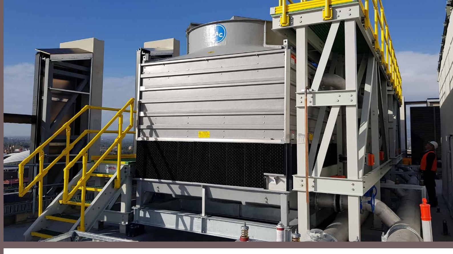
ArchitEX<sup>™</sup> FRP Structural Profiles are available in Isopthalic, Vinylester and temperature, fire resistance, smoke and smoke toxicity requirements must be taken into account, and will dictate which resin system is best suited for optimum performances over time.
